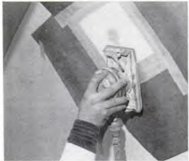
IF YOU HAVE a vibrating sander, use it. Start with 220-grit paper, wash sanded area frequently with water as you work to keep repair zone free of dust
